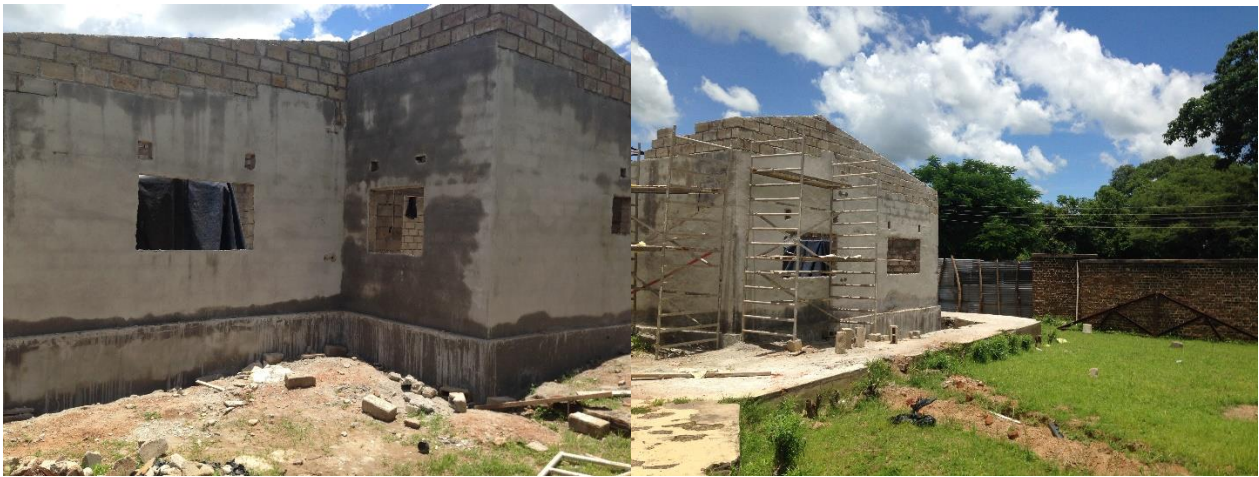
The oxygen plant house under construction
