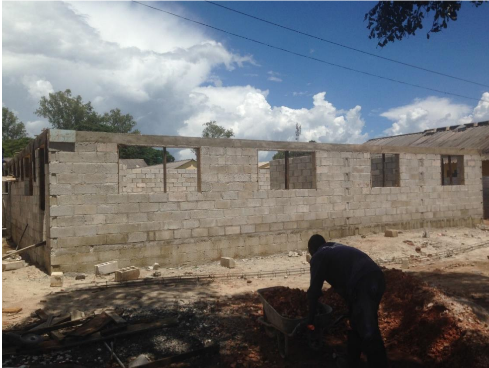
Physiotherapy building at construction
