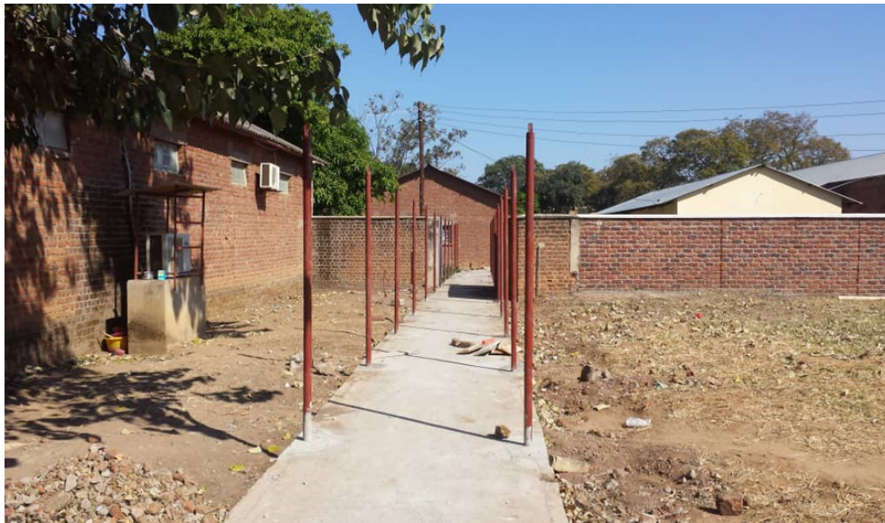
Roofing of walkways in progress
